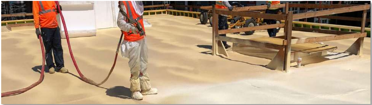
Pre-applying Silicone coating to curbs, penetrations, etc.
