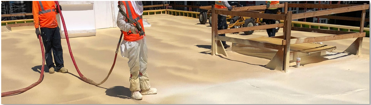
Pre-applying Silicone coating to curbs, penetrations, etc.
